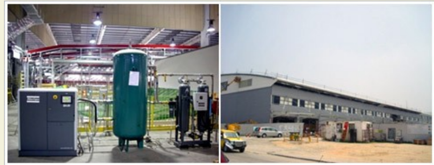
Design, Supply and Installation of Compressed Air System 設計、供應及安裝壓縮空氣系統
