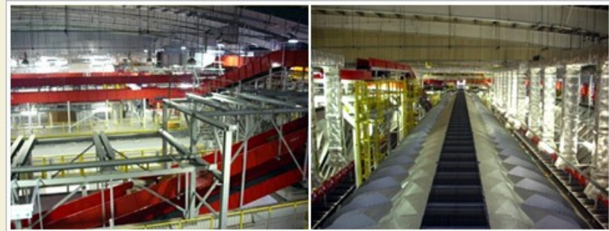
Installation and Modification of Sorter and Conveyor Systems 安裝及改裝運輸帶系統
