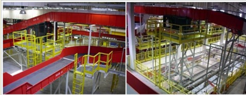
Design, Fabrication and Installation of Maintenance Platform 設計、製造及安裝維修平台
